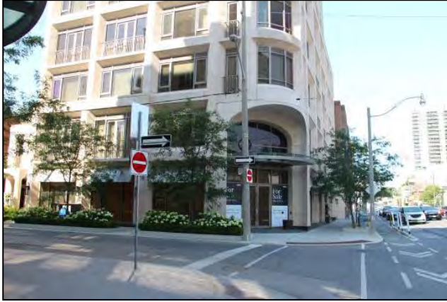
130 Hazelton Avenue Entrance
