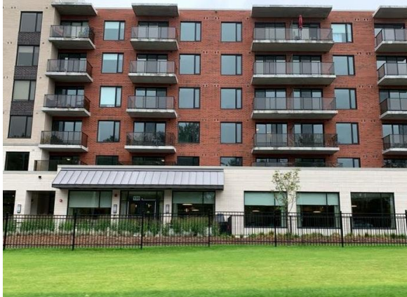
Existing Improvements - Exterior
