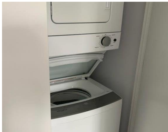
Typical Suite Finishings
