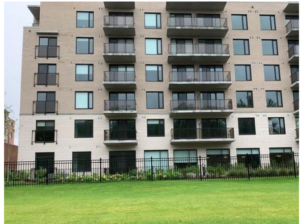
Tenth Line Road Frontage - Exterior
