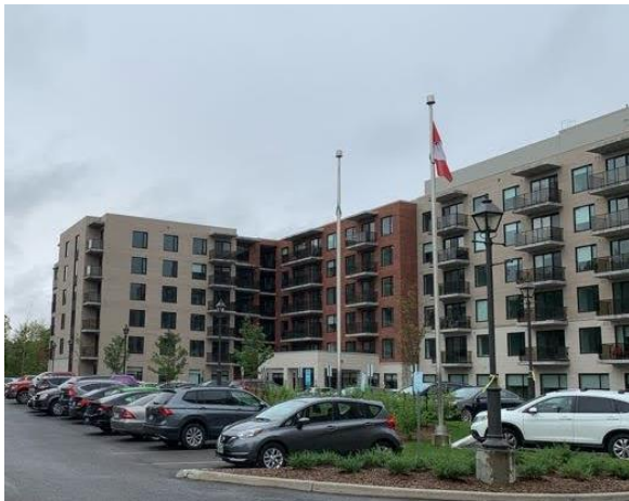
Exterior of Improvements
