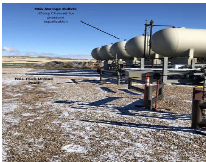
Figure A-6: The daisy-chained NGL storage bullets
