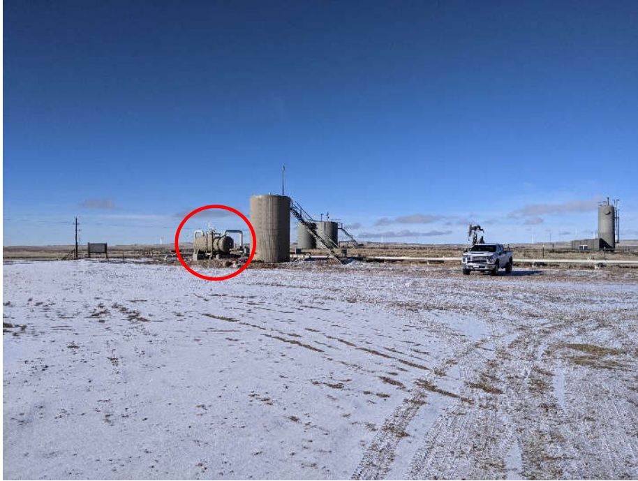
Figure A-3: The associated gas flows into this knock-out tank, circled in red, to separate any free water that didn't get removed at the well batteries
