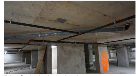
P3 – Sprinkler branch is in progress.
