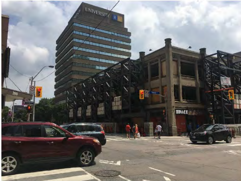
View from Gerrard Street
